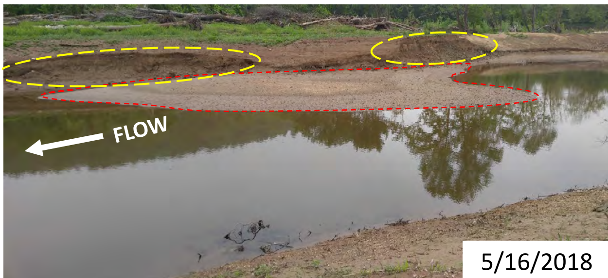
Figure 6. Deposition of fine sediment within trap; during low water (Pic: J.Collum)
