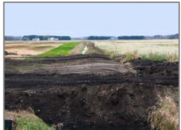
Figure 12. Finished Ditch Plug with Crown in Middle
