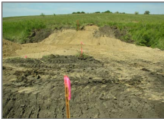
Figure 10. Ditch Plug under Construction
