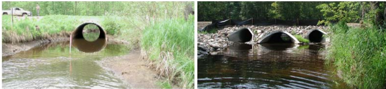
Undersized culvert.
