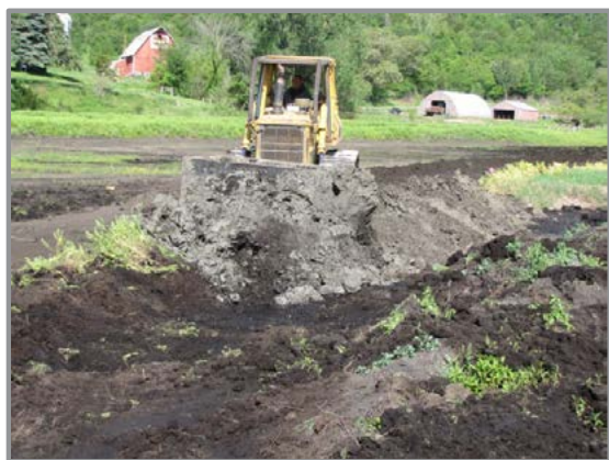
Figure 2. Shallow Ditch Being Filled
