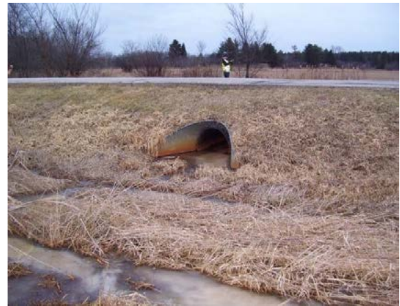
Concentrated Flow Entering Culvert Leading to Gully #7
