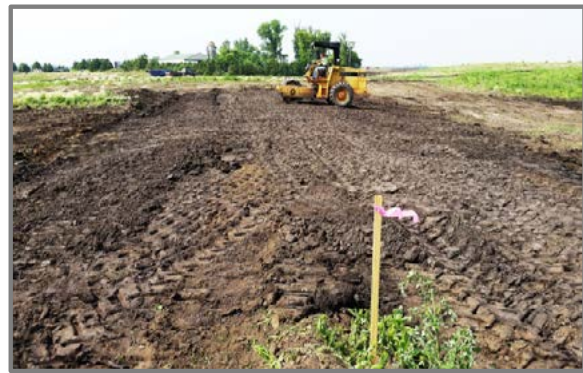
Figure 11. Compaction of Constructed Ditch Plug
