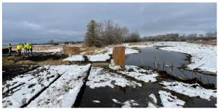
Before "tie in" of new channel with original channel: road plates divert water away from sensitive areas through a diversion channel.
